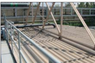
Tuff Span truss-supported cover
