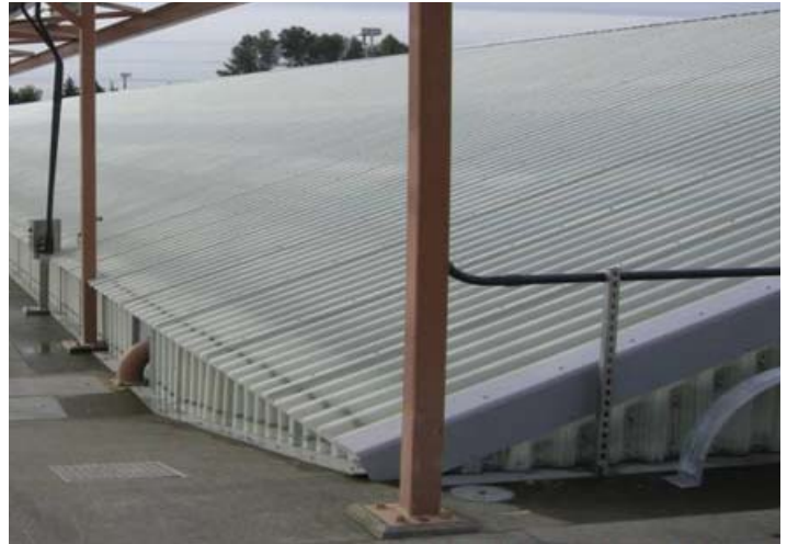
Tuff Span walk-in tank cover system with FRP translucent panels, beams, platforms and doors. Left photo shows the inside and right photo shows the outside. Aeration Basin
