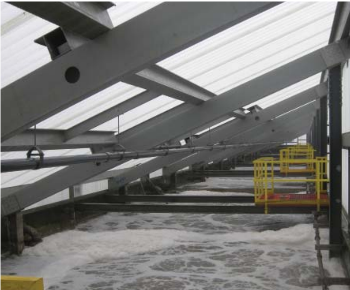
Tuff Span walk-in tank cover system with FRP translucent panels, beams, platforms and doors. Left photo shows the inside and right photo shows the outside. Aeration Basin
