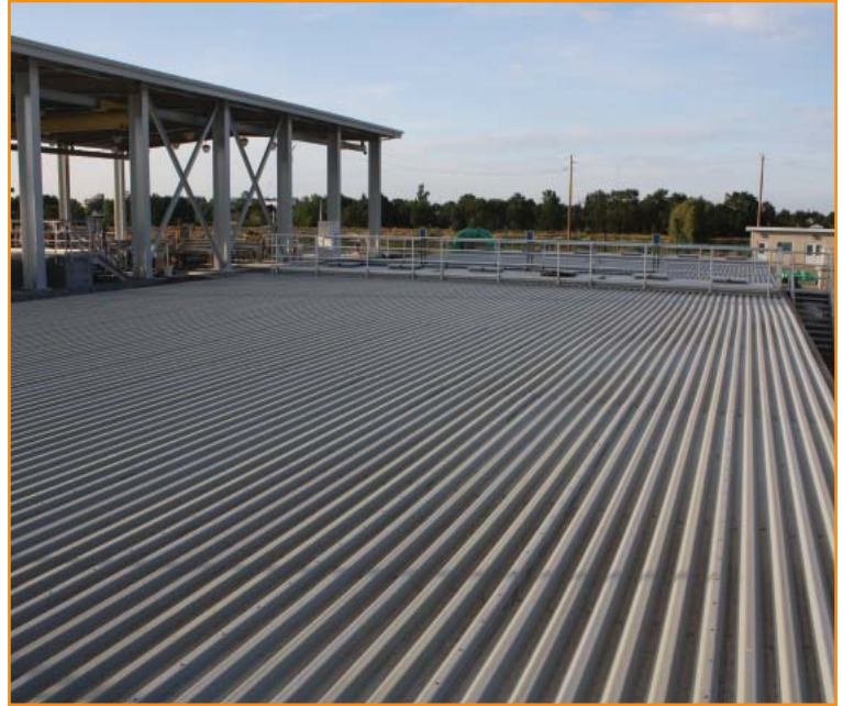
Tuff Span low-profile tank cover system with FRP beams UV Disinfection Process
