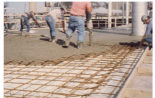
Tuff Span Form Deck at food processing plant.
