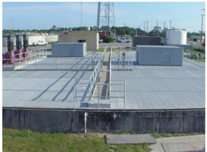
SureGrip beam-supported cover with Tuff Span removable enclosure. See pg. 13 for more about Tuff Span enclosures. Aeration Basin
