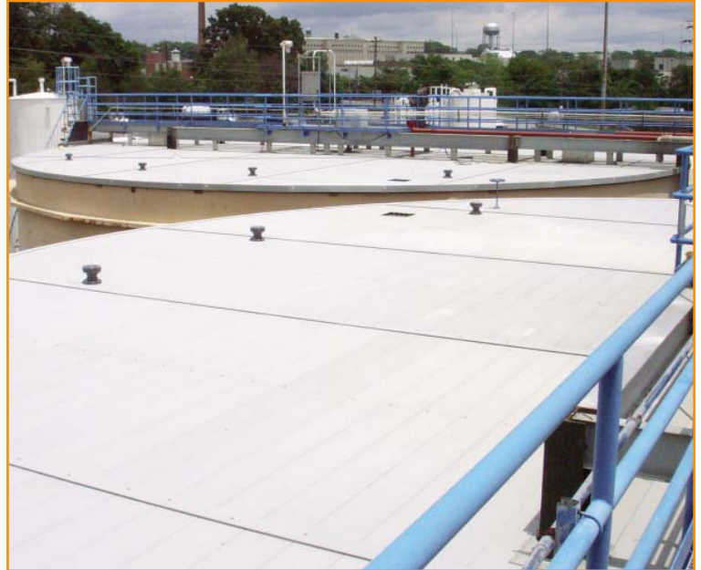
SureGrip beam-supported cover system over 70' diameter steel tank Aeration & Equalization Basin
