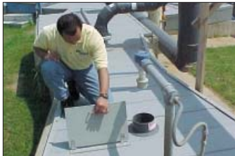
Viewports are lower cost and provide quick viewing.
