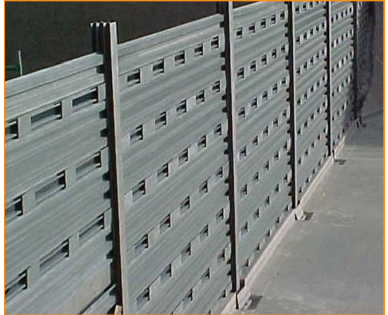
Enduro "H" slotted flow-thru baffle wall system Settling Basin
